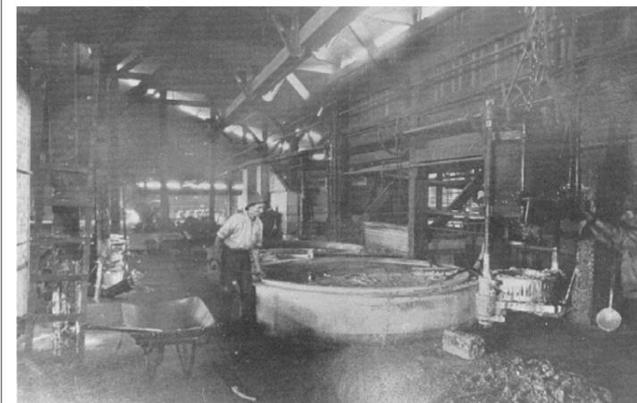
*Zinc being separated from tailings at BHP’s plant, by the Potter-Delprat process. Flotation technology developed in Melbourne and Broken Hill a century ago is economically Australia’s most significant contribution to industrial technology.*
