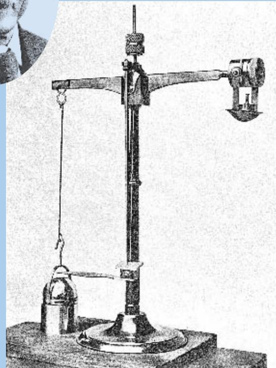
*A ball and socket viscosimeter—an apparatus invented by A.G.M. Michell in 1919 for measuring the viscosity of lubricants.*
